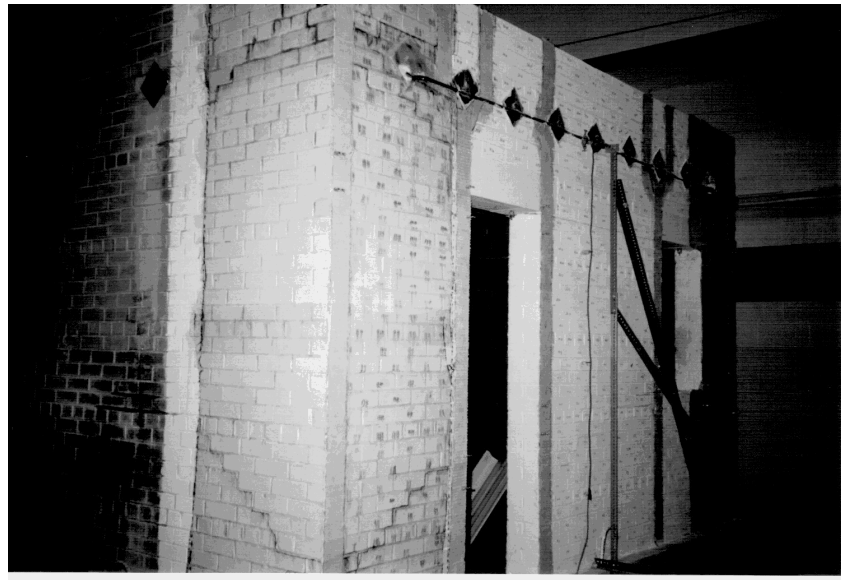
Figure 7: URM specimen repaired with Tyfo material (strips and web)
