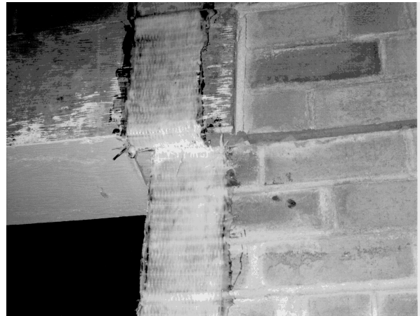
Figure 10: Tyfo strip failed in shear
