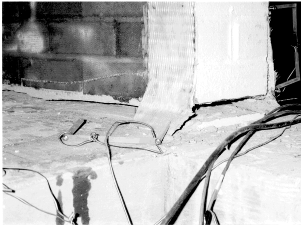
Figure 9: Pier rocking at large displacement
